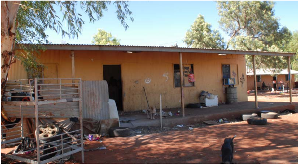
ABOVE: Bessie and Jeffery's two-bedroom corrugated iron house with no insulation. It is freezing in winter, when overnight temperatures fall below 0°C, and unliveable in summer, when daytime temperatures reach 45°C. Eleven people live in this house. © Al/Lucas Jordan
