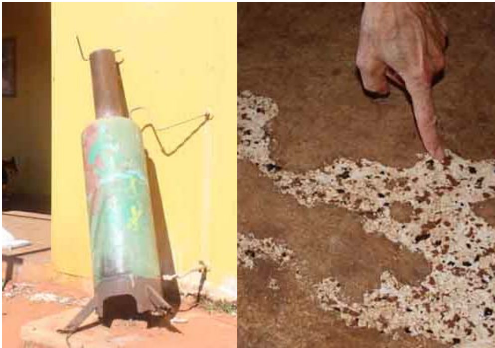
BELOW RIGHT: Chipboard inappropriately installed as flooring, easily damaged and affected by rising damp. © Lucas Jordan/AI
