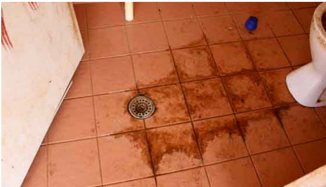
ABOVE: Ongoing sewerage problems including effluent overflow in shower recess, bathrooms and toilets due to blockages. © AI/Lucas Jordan
