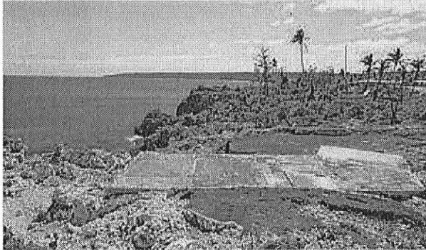
Niue: what's left of the community centre. Many trees are missing and those still standing have been stripped not only from their leaves but from their branches as well. 2
